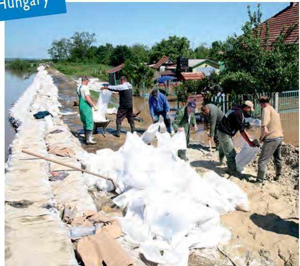
Despite the heroic efforts by the community, the flood caused considerable damage
