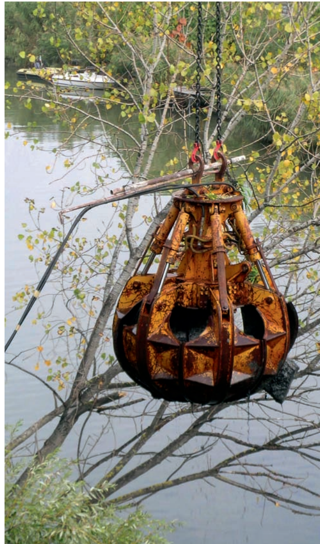
Removing the rubble near the Ponte Nuovo at the far end of the river will help restore the natural flow.
