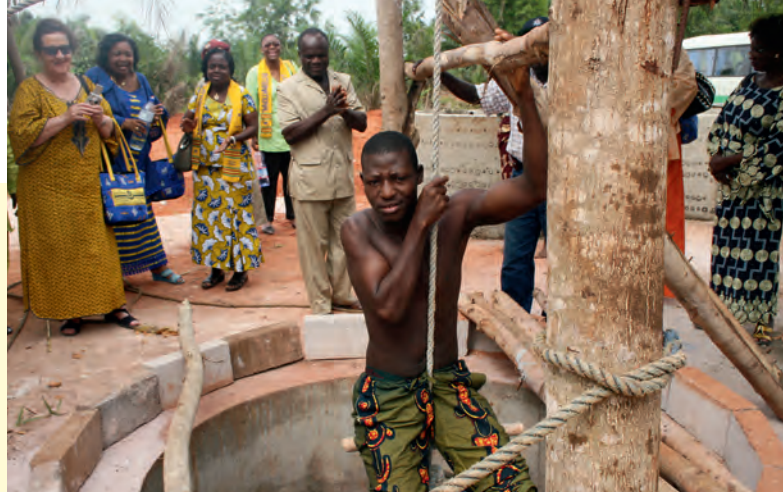
This well in Dangbo is 60 metres deep and was constructed with limited technical means.
